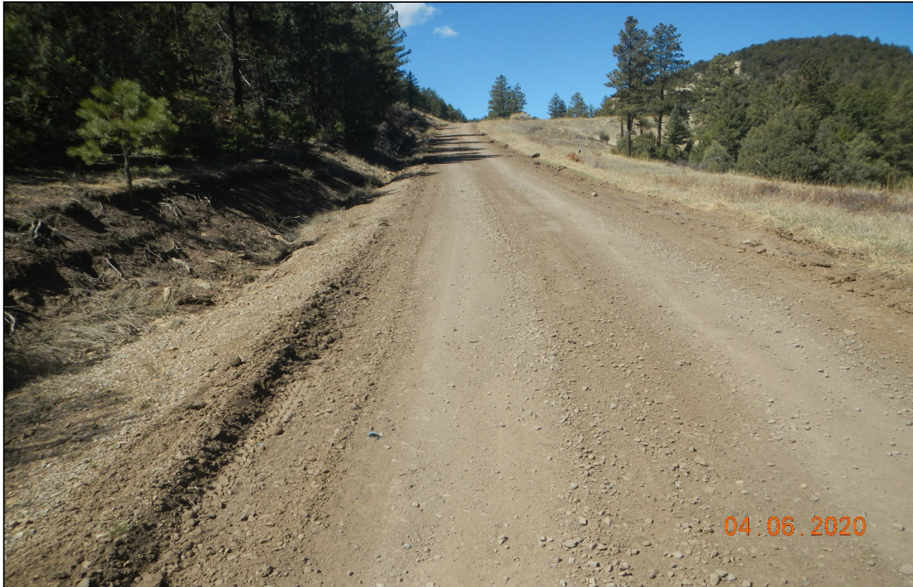
Photo 2. Facing northwest along the main lease road toward the location. The road has graded.
