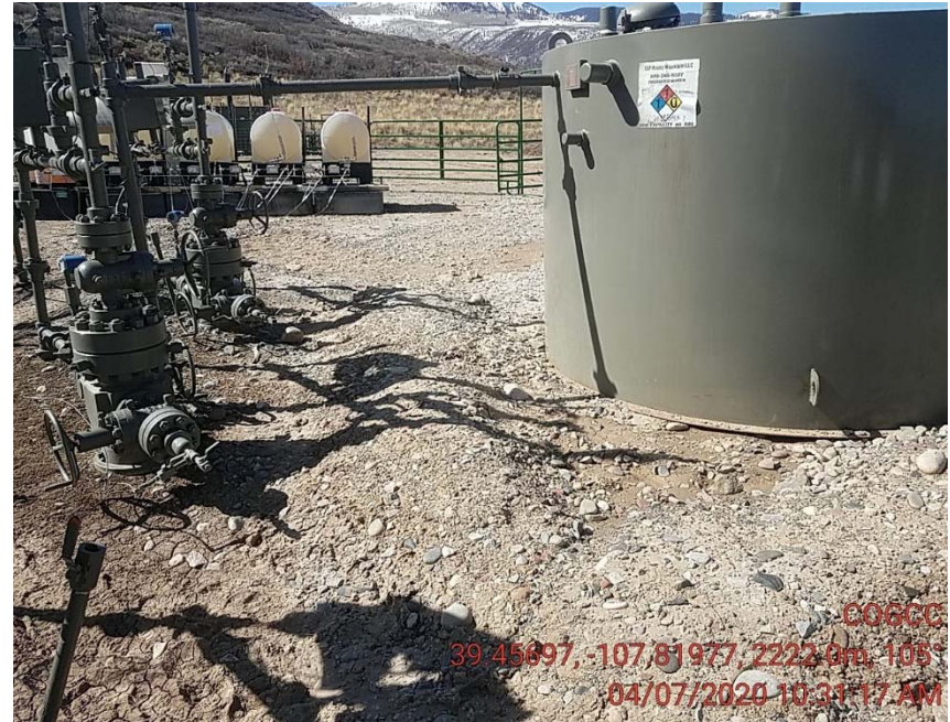
Lack of secondary containment
