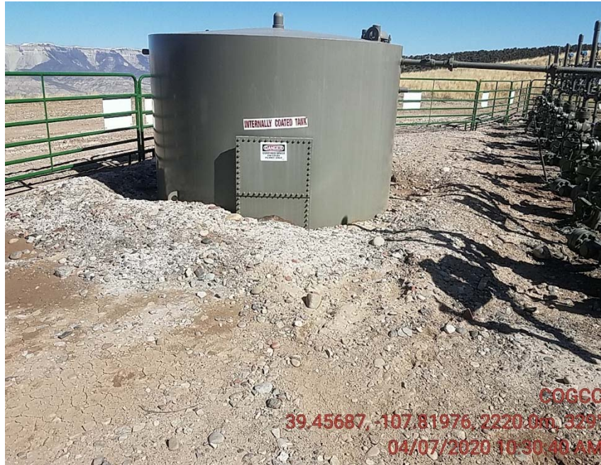
Lack of secondary containment
