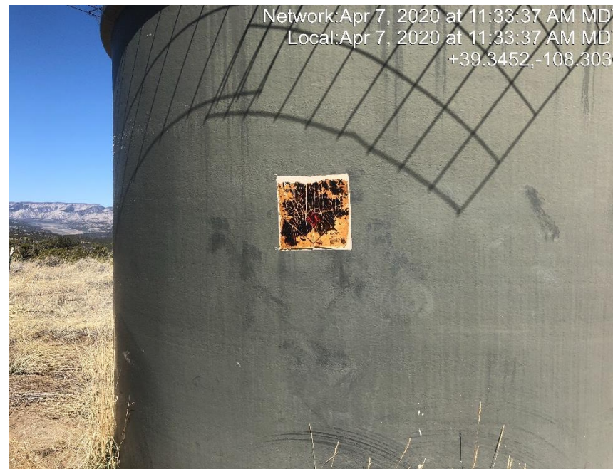
Photo #0921 Tank NFPA label weathered and not legible.
