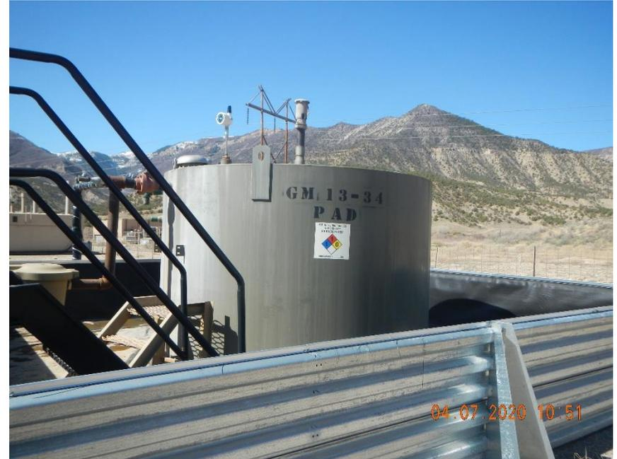
**No tank capacity on production tank.**
