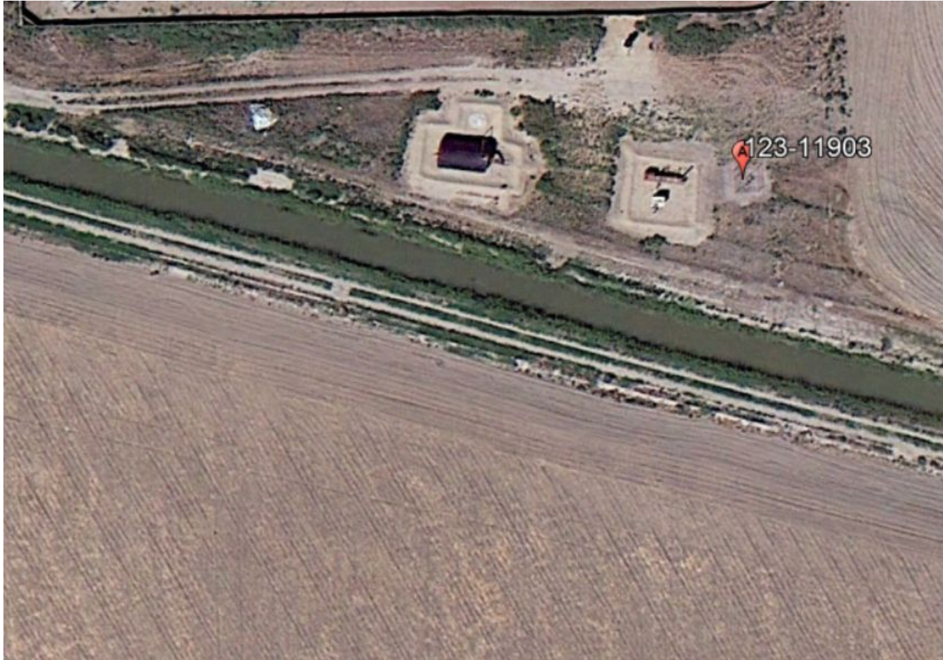
Photo 1. Google Earth aerial imagery taken 8/18/2012 during active operations illustrates the disturbance areas.
