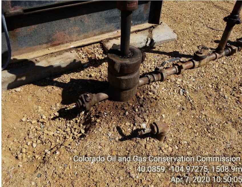
Photo 3 stained soil around well head
