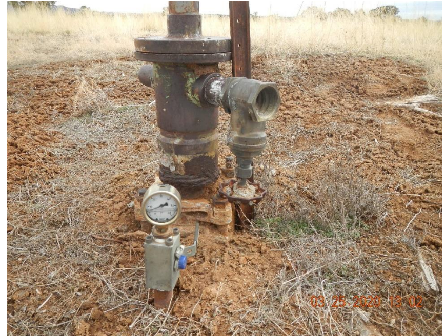
PA well head. Concrete can be seen in tubing and production strings. Bradenhead valve access with valve closed.
