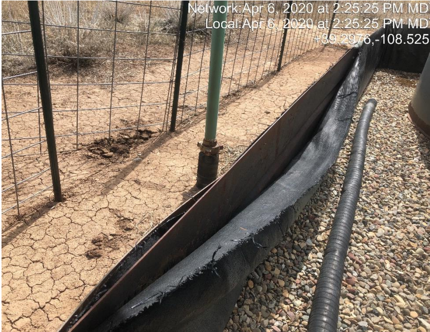
Photo #0914 Tank containment liner in need of maintenance.
