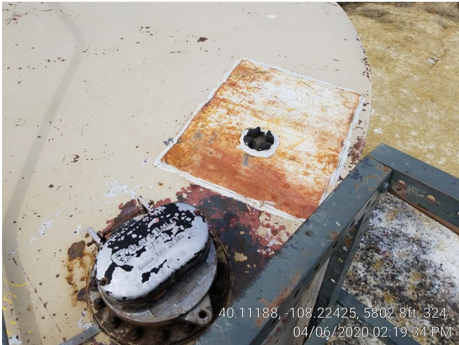
Photo 5. Top of tank patch.
