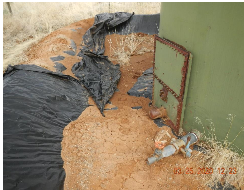
Compromised liner on secondary containment berm.
