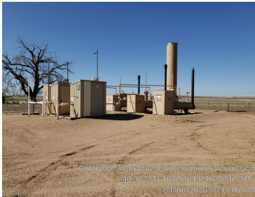
Photo #5 Separators, ECD & Meter Runs
