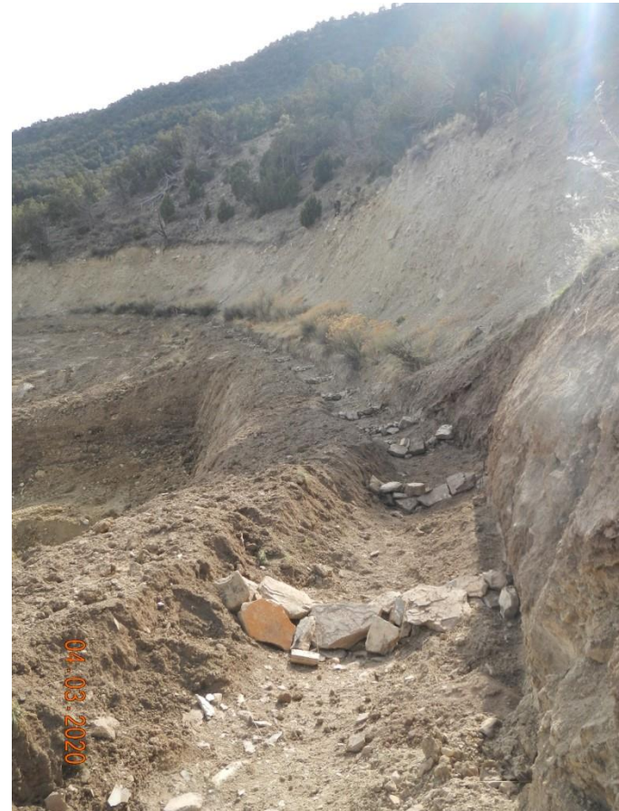
Photo#6: Ditch/check dams along West cut slope.
