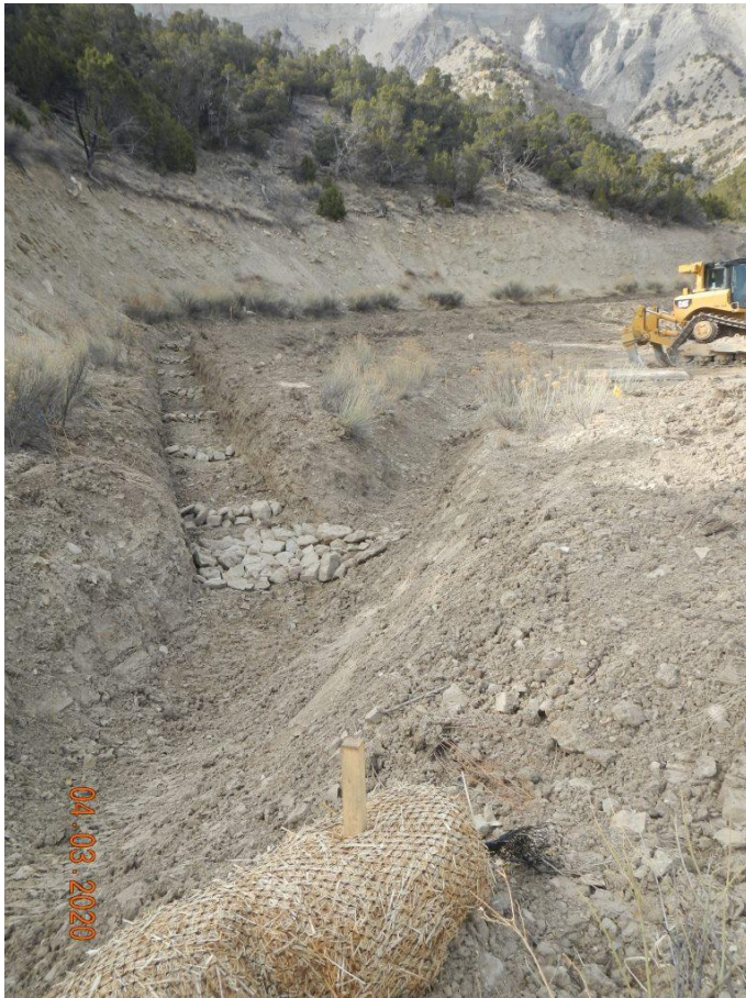
Photo#5: Ditch/check dams along West cut slope.
