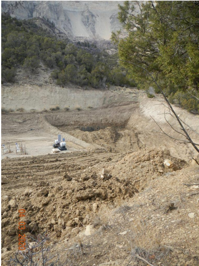
Photo#8: View of pit excavation from East Cut slope, where material is being layered.
