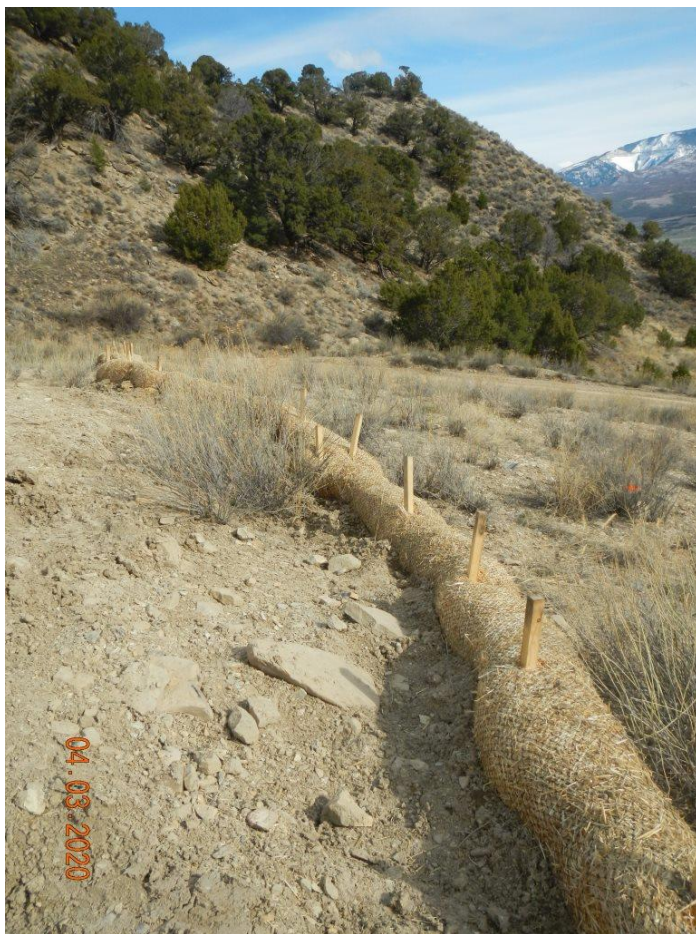
Photo#3: Wattles installed at perimeter.
