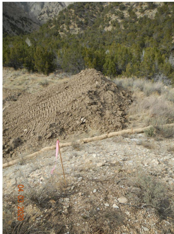
Photo#4: Wattles at presumed Topsoil Pile.
