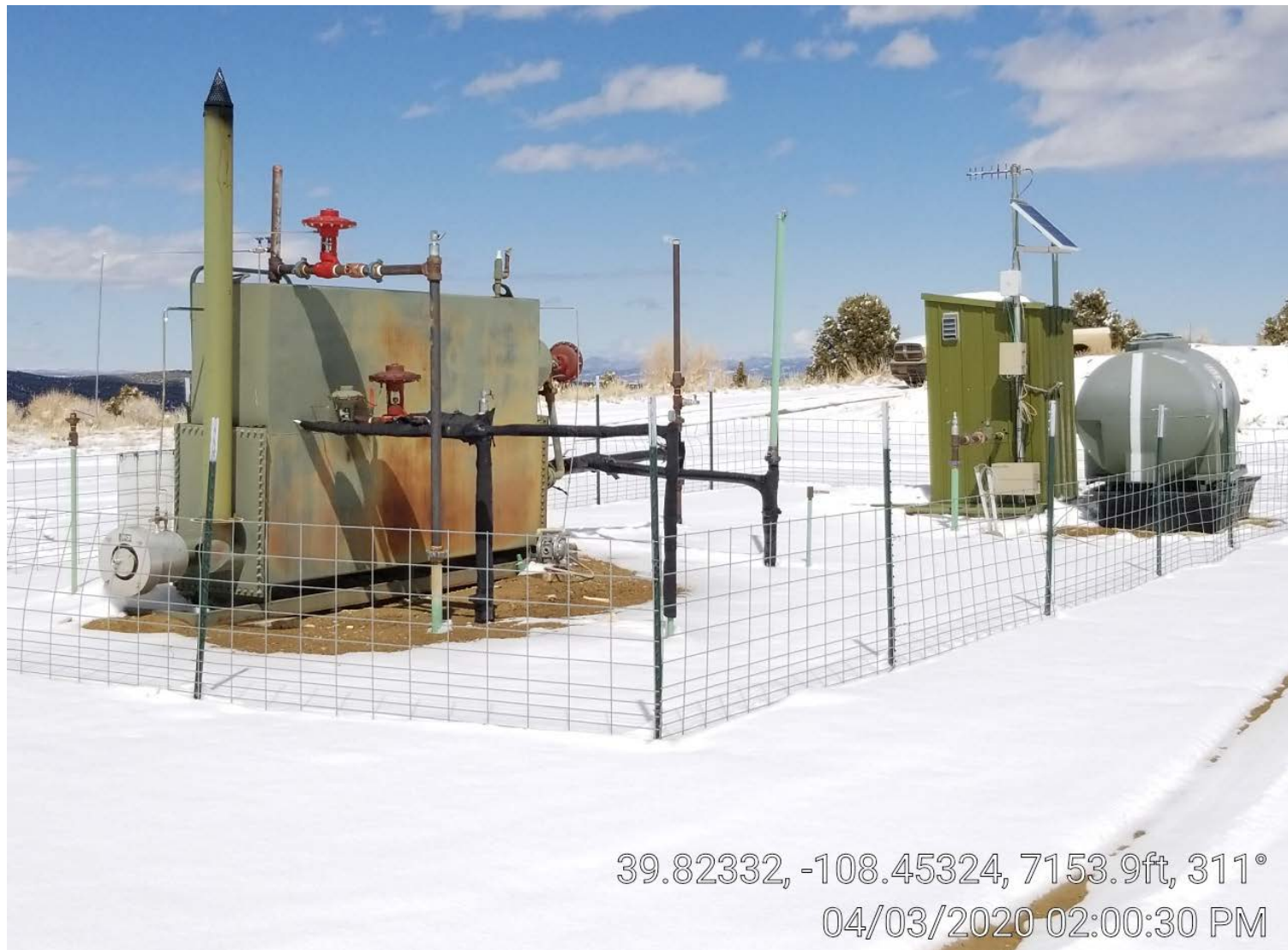
Photo 3. Separator & meter building.
