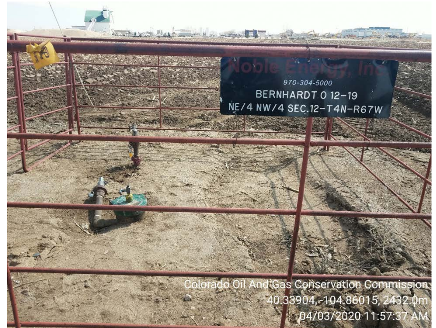
Unused equipment on 4/3/2020
