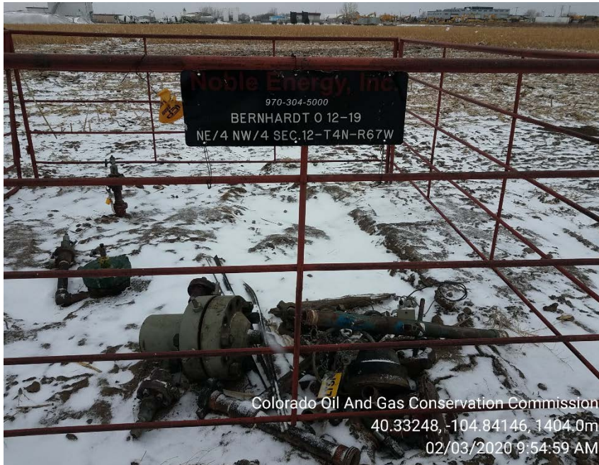
Unused equipment on 2/3/2020
