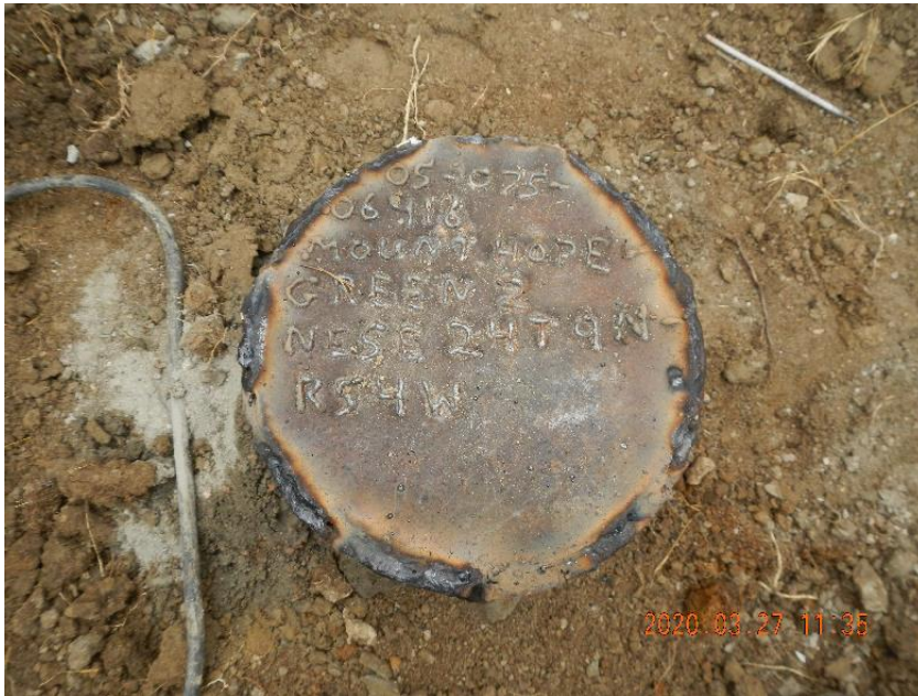
Photo 7: Marker plate welded onto surface casing.
