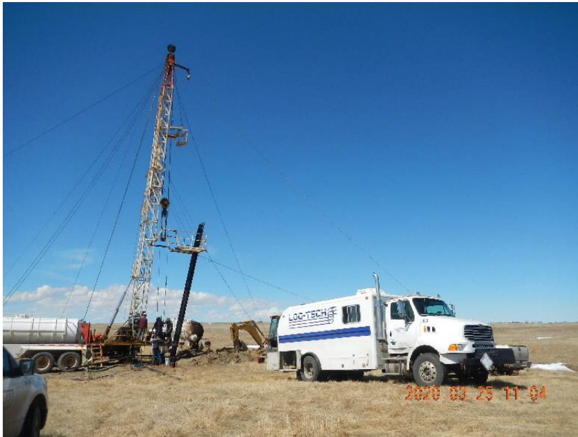
Photo 3: Wireline on location to run CBL, perforate well for cement plugs, and set CICR.
