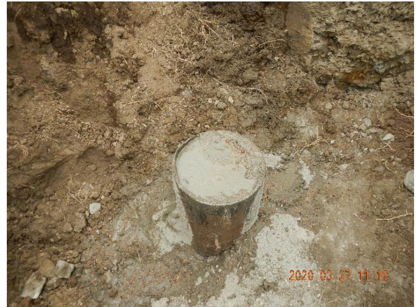
Photo 6: Surface casing topped off with cement.
