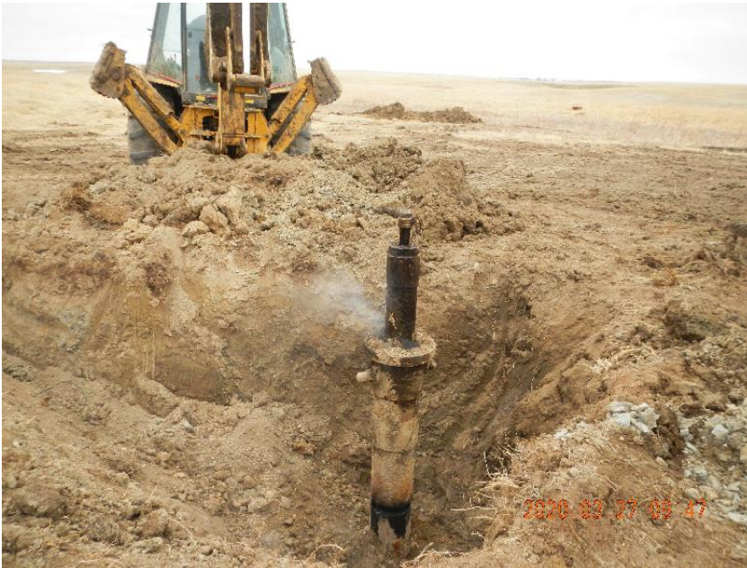
Photo 5: Excavated surface casing.
