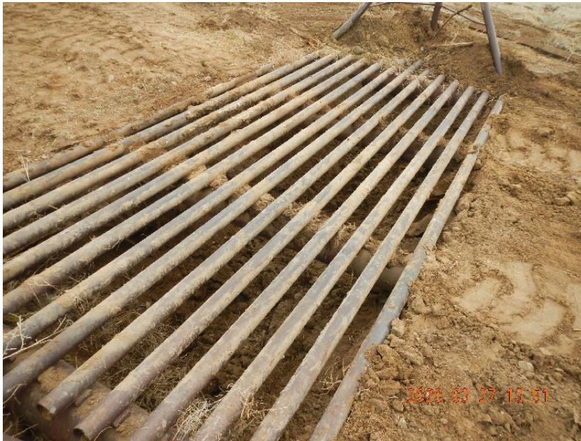
Photo 13: Center depth view after clean out.
