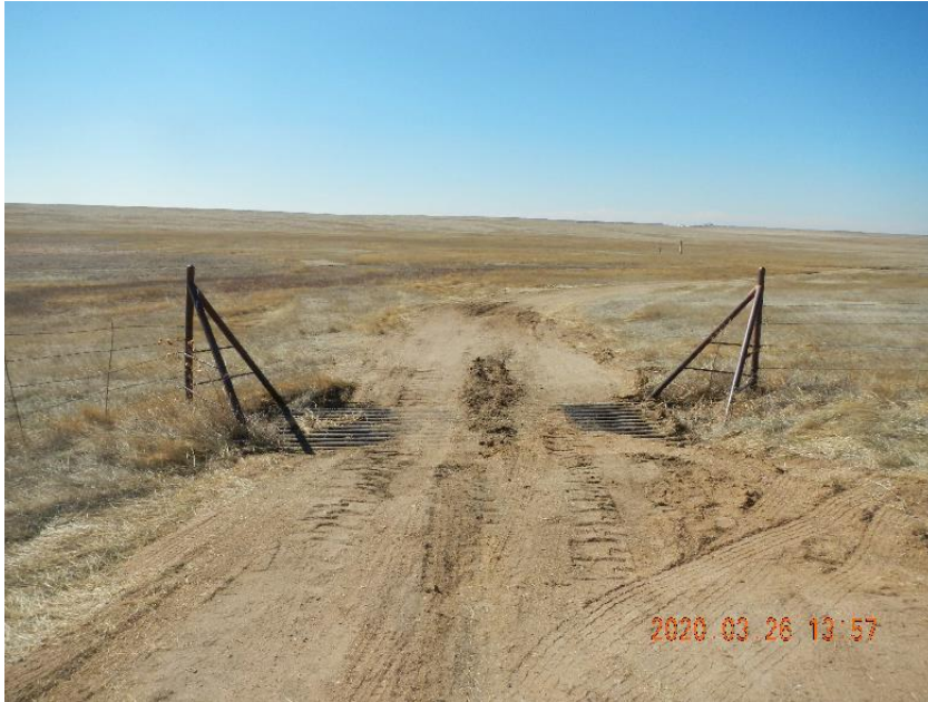
Photo 11: View of cattle guard at access entrance before clean up.
