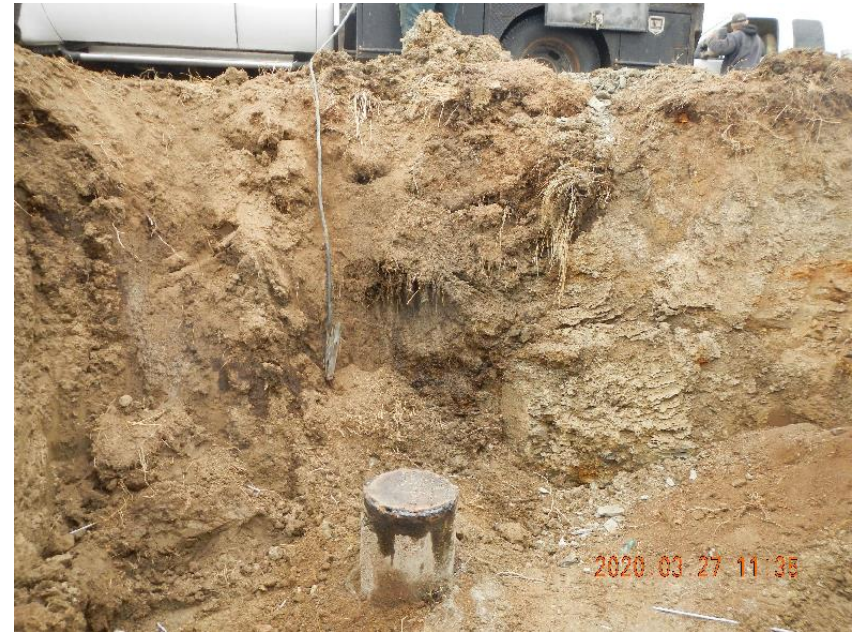
Photo 8: Surface casing ready for backfill.
