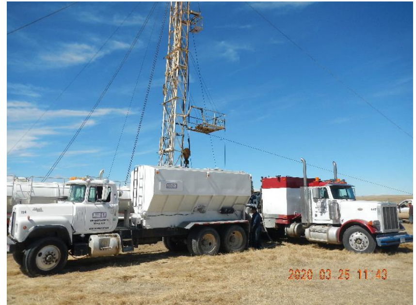
Photo 4: Cement equipment on location to pump cement plugs.
