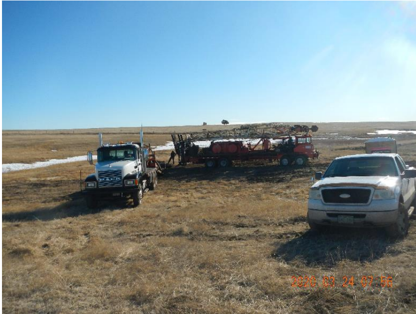
Photo 1: Spotting equipment in at well.
