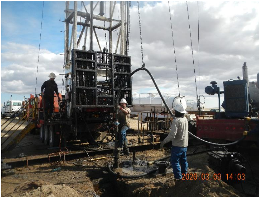
Photo 7: Rigging up to pump surface plug.
