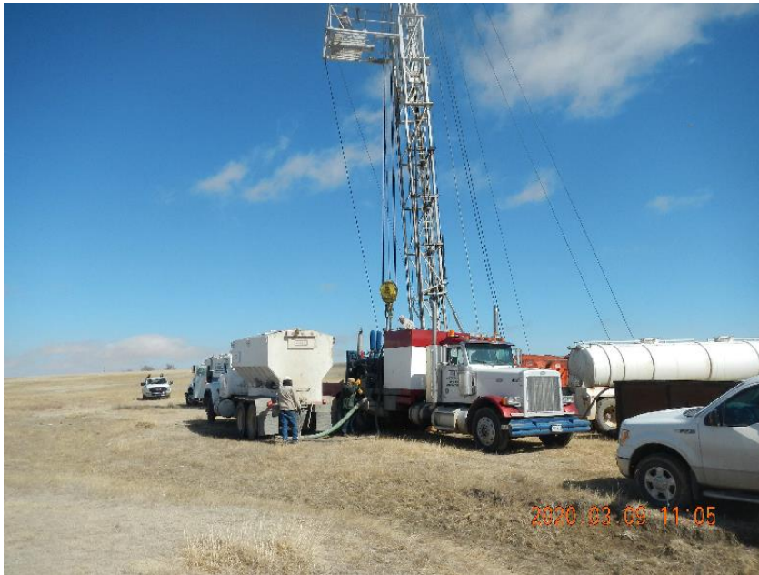
Photo 5: Cement pump truck rigged into well to pump cement plug.
