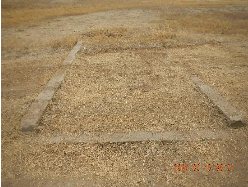
Photo 15: Possible cattle guard along access road.
