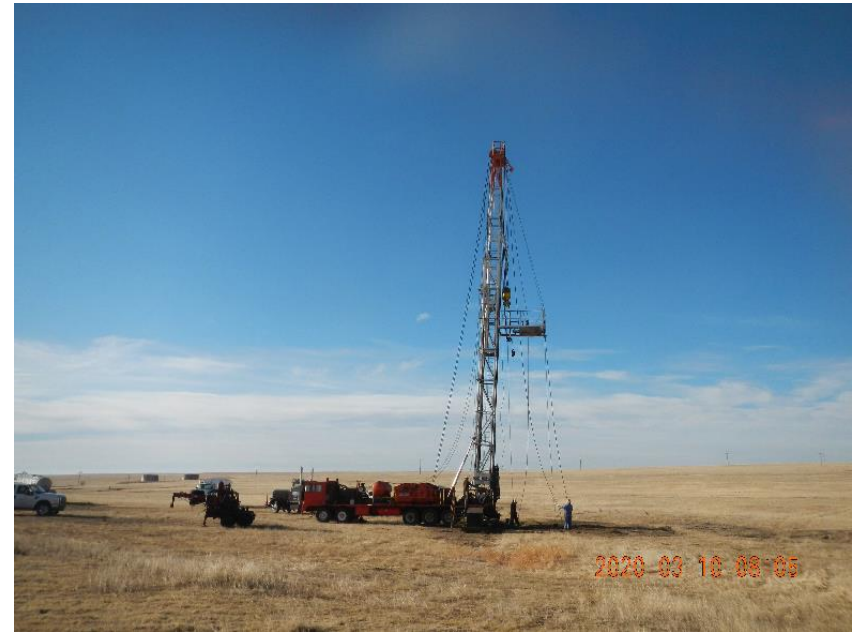
Photo 8: Rigging down to move.
