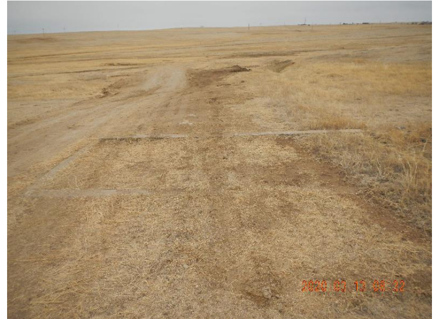
Photo 16: Access road with cement base along right side of road.
