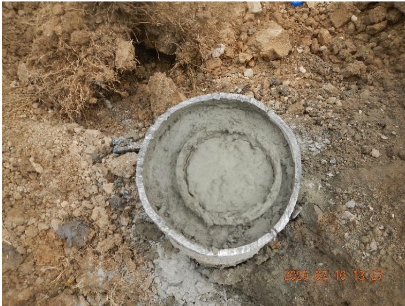
Photo 9: Surface casing topped off with cement.
