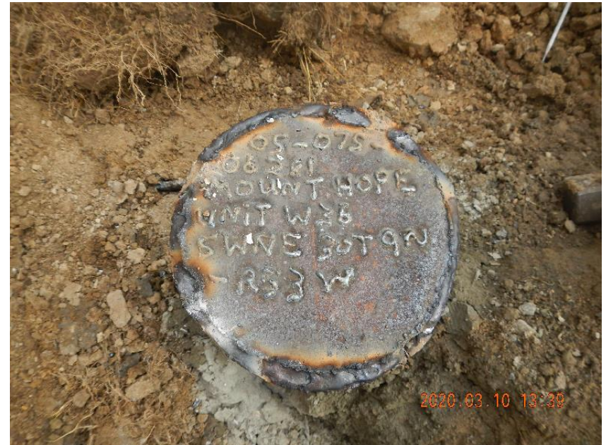
Photo 10: Marker plate welded onto surface casing.
