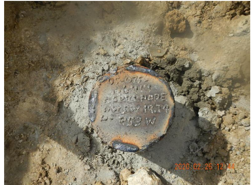
Photo 10: Marker plate welded onto surface casing.
