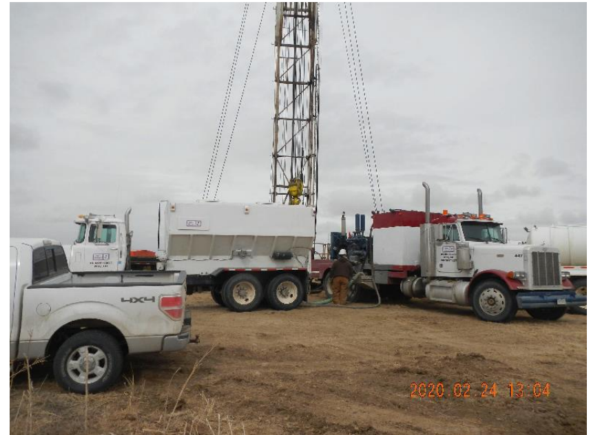
Photo 4: Cement equipment rigged into well to pump cement plug.
