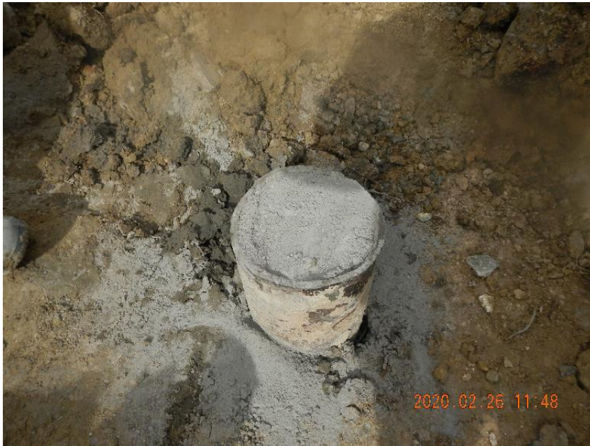
Photo 9: Surface casing topped off with cement.
