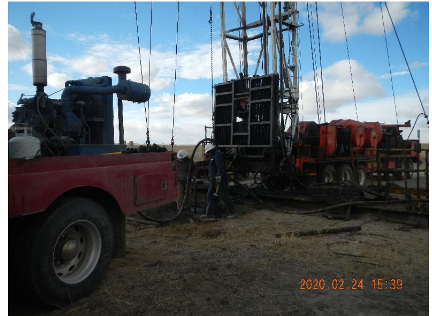
Photo 8: Setting up to bullhead surface plug.
