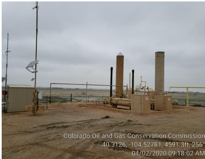
Photo #1 Separators, ECD's & Meter Run
