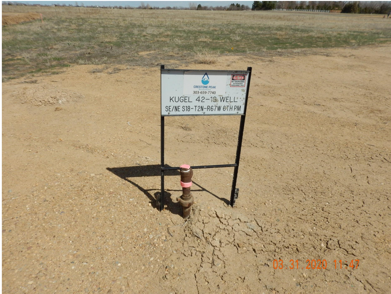
Photo 1. Photo taken from the Kugel 42-18 well location, facing North. Photo illustrates Operator has failed to remove a riser per Rule 1004.a.
