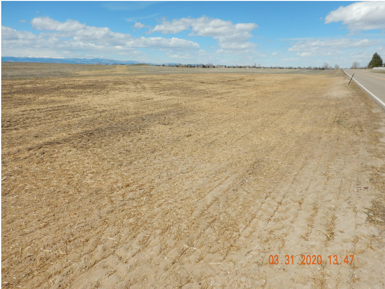
Photo 5. Photo taken from the associated offsite tank battery location, facing North. Photo illustrates Operator has removed all equipment and has performed final reclamation activities with the evidence of drill rows and straw crimped mulch.
