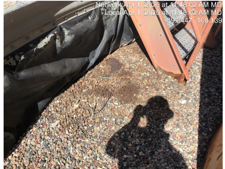
Photo #0893 Stained gravel inside tank containment.
