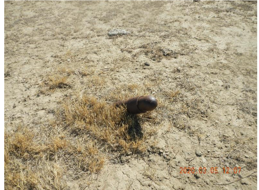
Photo 6: Close up view of flowline.
