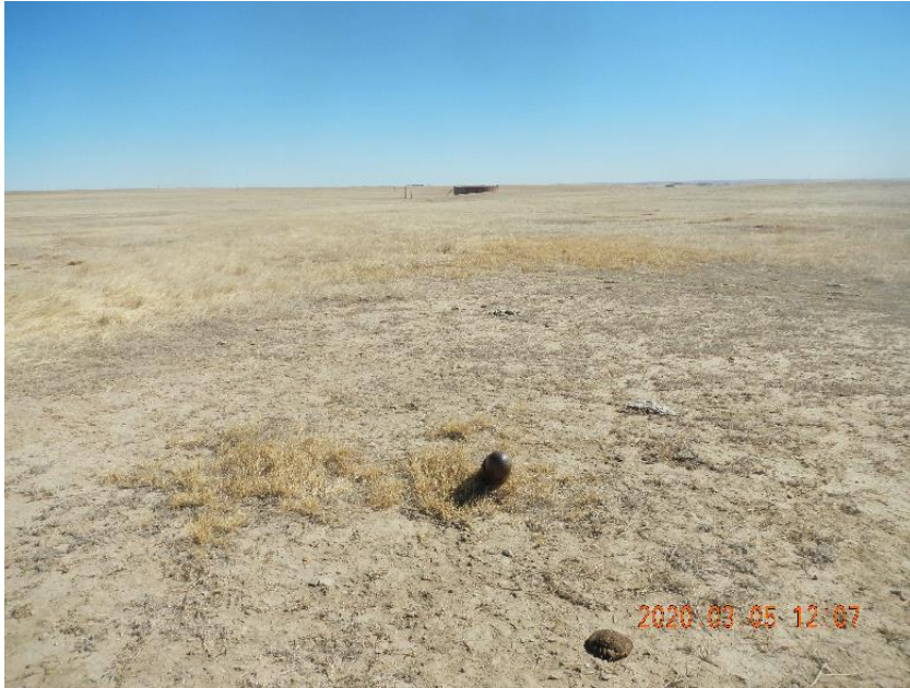
Photo 5: 3" flow line with 5000 BBL tanks in background.
