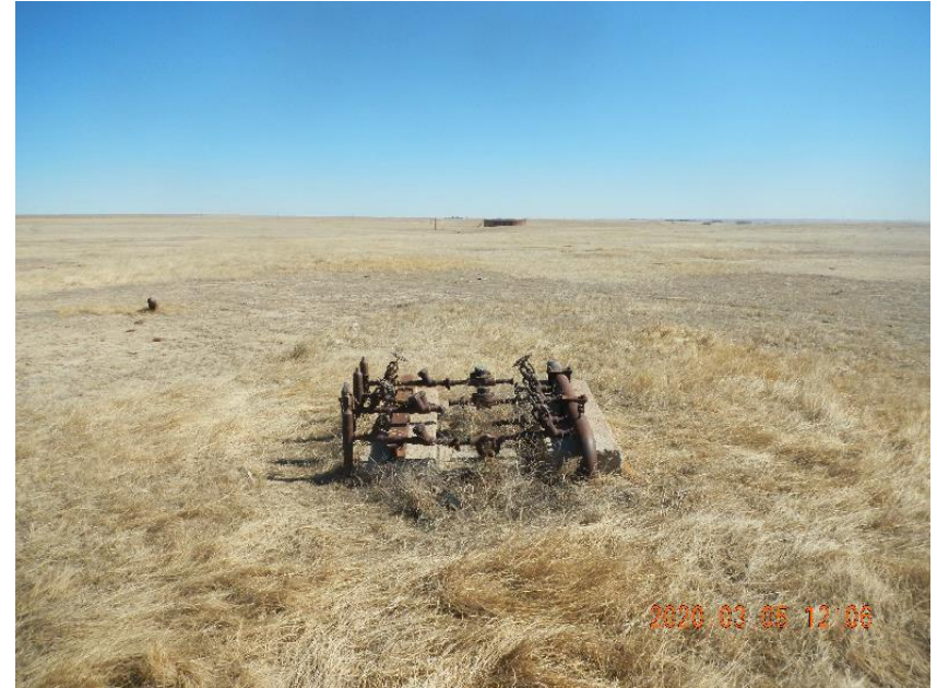
Photo 4: Header with 5000 BBL tanks in background.
