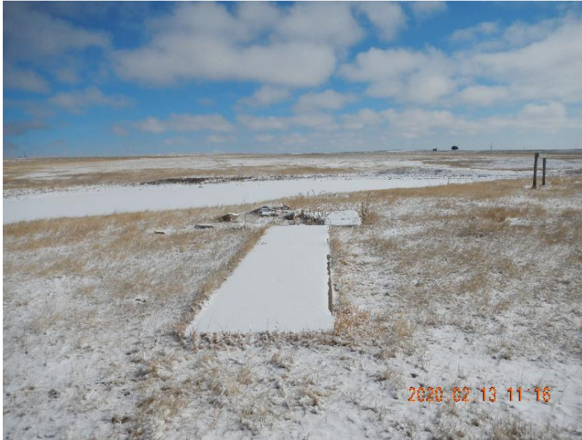
Photo 1: Concrete slab appears to be 6" - 8" thick.
