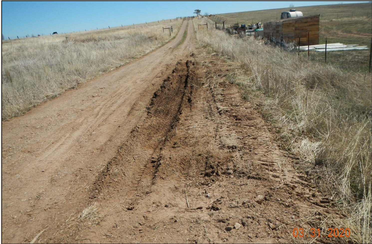
Photo 4. View of area along the access road where water is ponding and deep mud is resulting in expansion of road disturbance and rutting.
