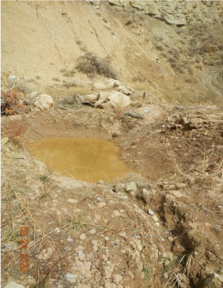
Photo#3: BMP at North end of site needing maintenance.
