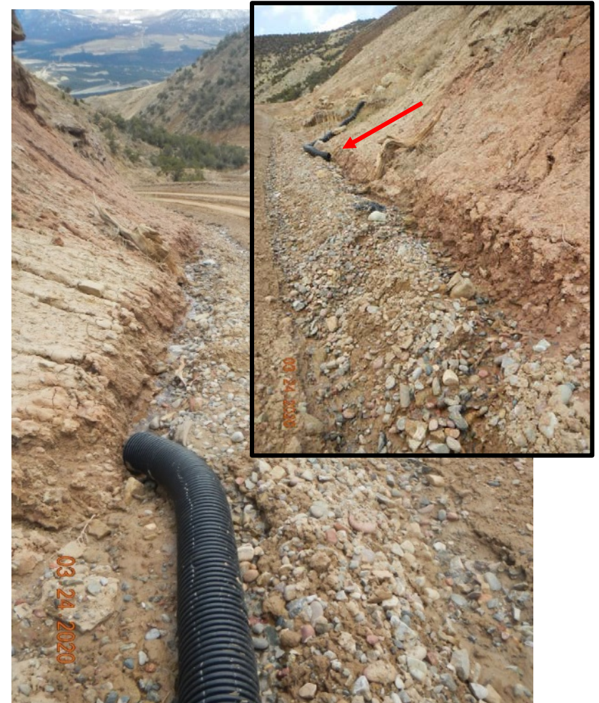
Photo#17: Flexible drain discharge point into access road ditch.
