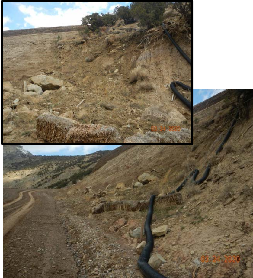
Photo#16: Flexible drain to convey stormwater from pad above and BMP in Photo#14.
