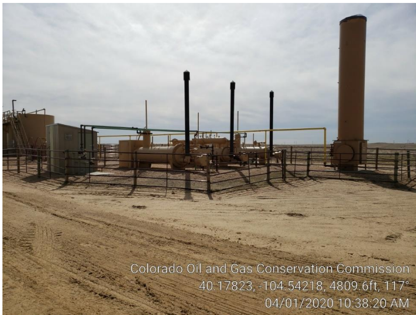
Photo #3 Separator's, ECD & Meter Runs
