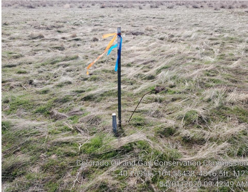
Photo #5 Marked Guy Line Anchor
