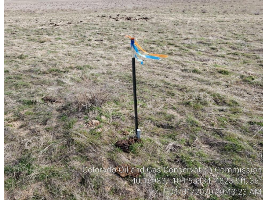
Photo #6 Marked Guy Line Anchor
