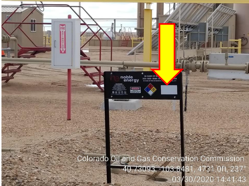
Photo 5 – Vault North of Compressors is missing Content and Capacity
