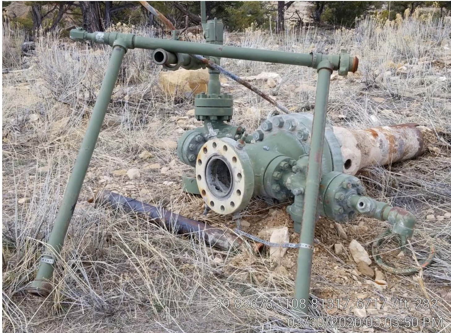
Photo 3. Well head from P&A well.
