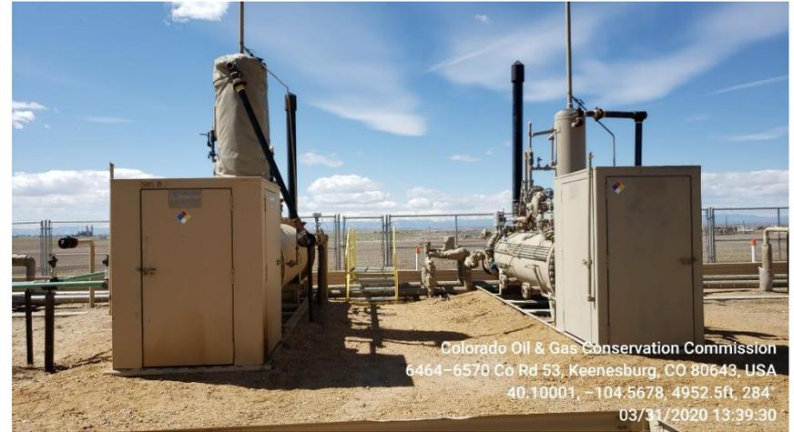
**Photo 5 Verticle Separator**
