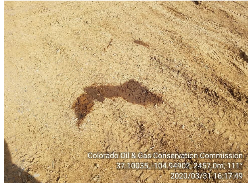
PHOTO 4: AREA OF IMPACTED SOIL BETWEEN WELLHEAD AND METER HOUSE. Conduct maintenance on equipment, cleanup stained material and review self inspection processes. CA DATE 4-30-20.
