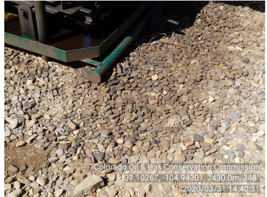
PHOTO 4: AREA OF IMPACTED SOIL APPEARS TO BE OIL CONTAMINATION FROM COMPRESSOR. Conduct maintenance on equipment, cleanup stained material and review self inspection processes. CA DATE 4-30-20.
