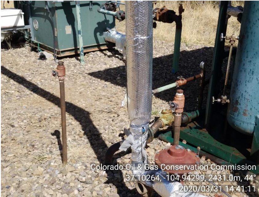
PHOTO 5: TWO UNMARKED UNUSED RISERS. COMPLY WITH NTO AND RULE 603.f. CA DATE 4-30-20.
