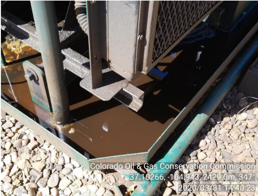
PHOTO 3: STANDING OIL IN COMPRESSOR SKID. COMPLY WITH GENERAL PERVISIONS OF OIL AND GAS ACT PERTAINING TO WILDLIFE PROTECTION. CA DATE 4-30-20
