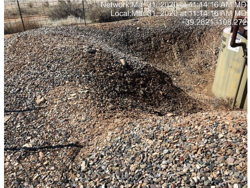
Photo #0879 Secondary containment berm has eroded.
