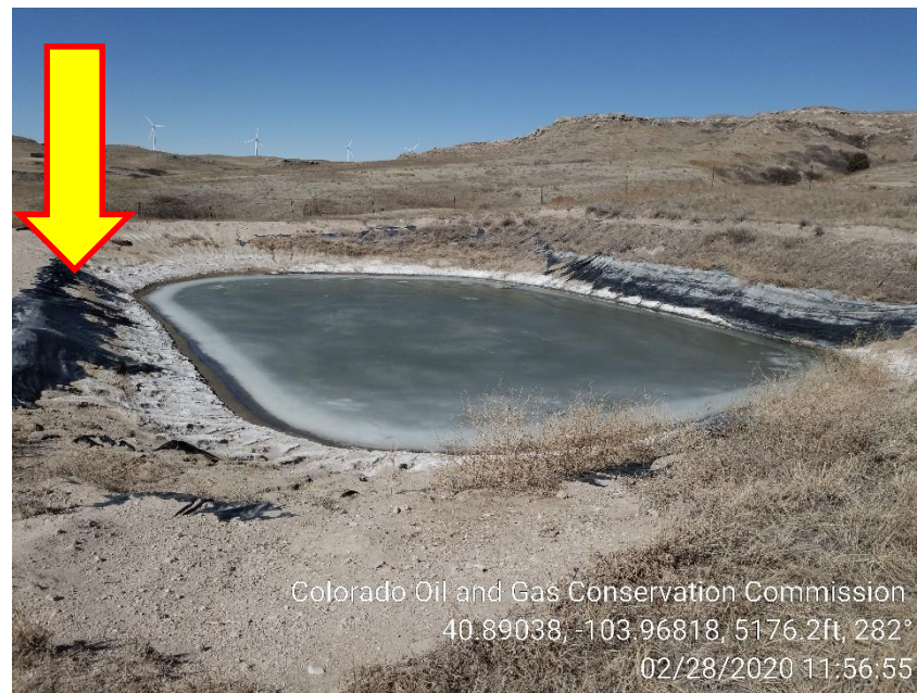
Photo 7 – NE Pit; holes in lining
