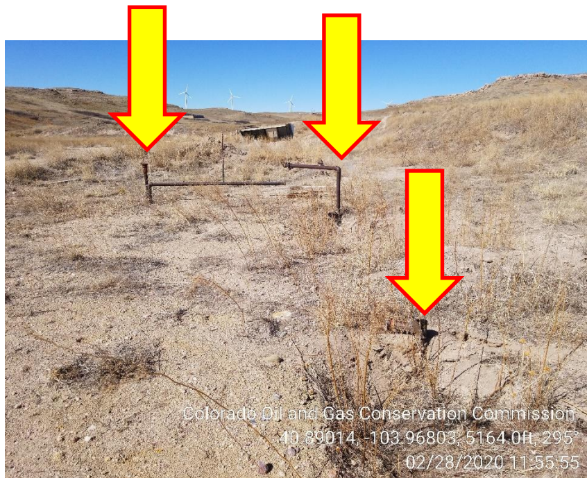
Photo 12 – Unmarked Risers
