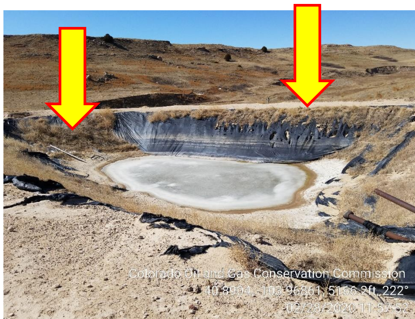
Photo 8 – West Pit; hole in lining and weeds
