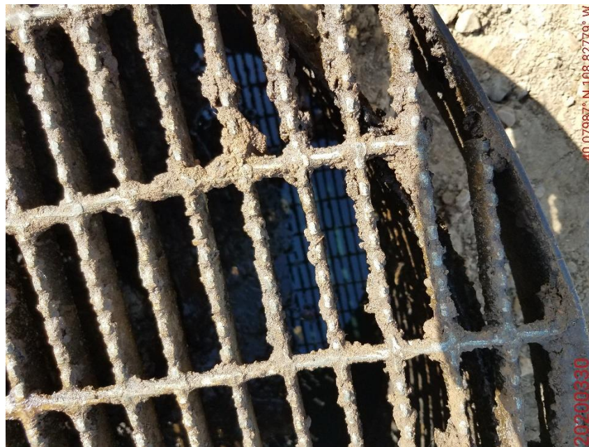
Photo 2: Photo of containment cellar at the wellhead. . Inspection #696201101 required Operator to remove fluids/chemicals within containment. Photo shows fluids/chemicals have not been removed per corrective actions.
