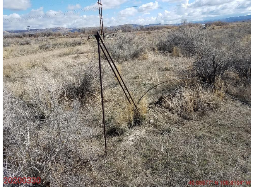
Photo 8: Continued from photo 7. Photo shows utility anchor and cable.
