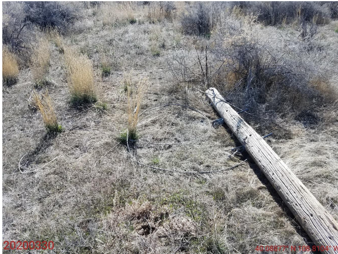
Photo 9: Continued from photo 7. Photo shows cut utility pole and cable wire.
