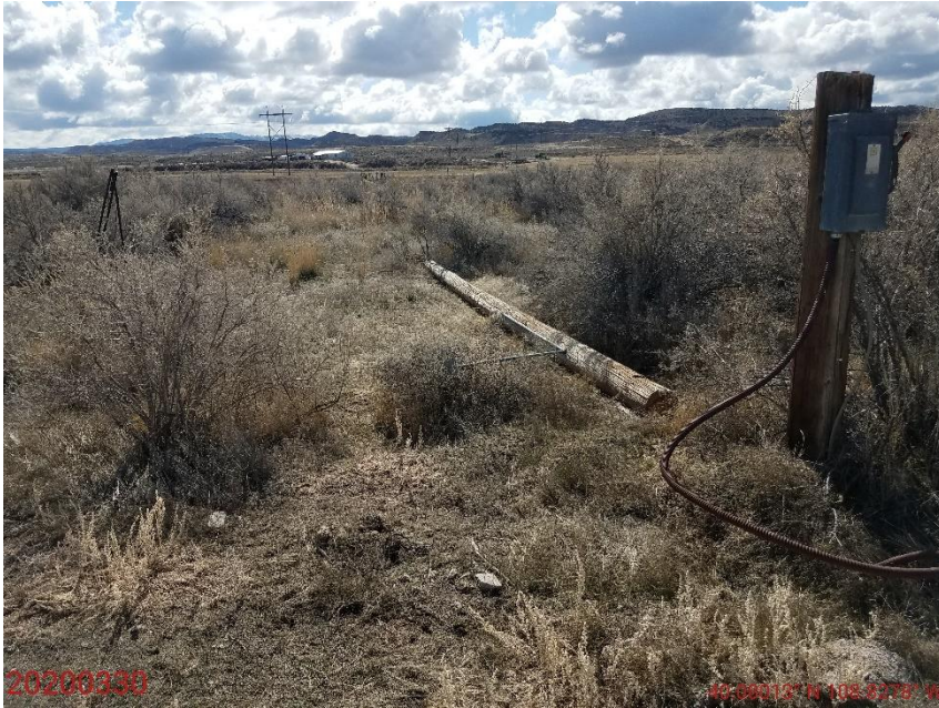
Photo 7: Photo taken from the southeast end of the Location, facing south. Photo shows the utility pole appears to have been cut above the electric box. Cut portion of the utility pole, as well as cable wires and the utility anchor was not removed, is considered unused equipment and trash debris, and requires removal.
