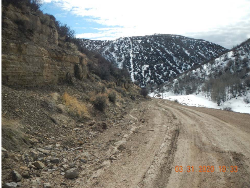
Photo 3. Sediment moving down access road and on left hand side of road.
