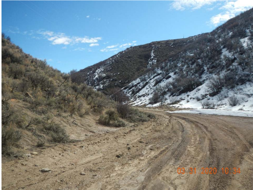
Photo 5. Sediment moving down and across access road into drainage.
