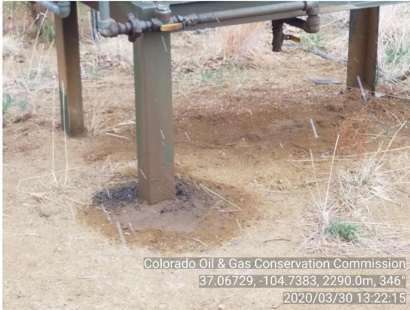
PHOTO 3: AREA OF IMPACTED SOIL APPEARS TO BE OIL FROM COMPRESSOR. Conduct maintenance on equipment, cleanup stained material and review self inspection processes. CA DATE 4-30-20.
