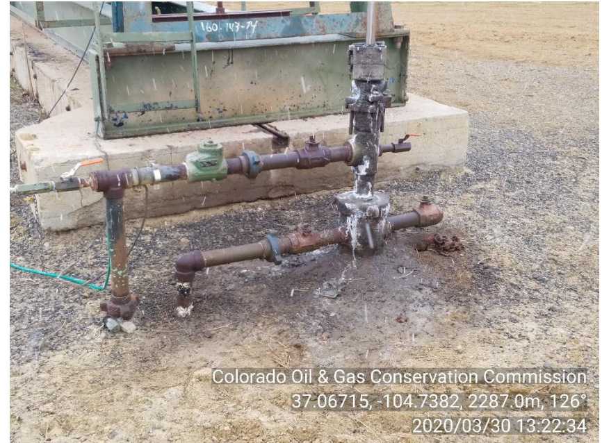
PHOTO 4: AREA OF IMPACTED SOIL APPEARS TO BE OIL FROM POLISH ROD LUBRICATOR. Conduct maintenance on equipment, cleanup stained material and review self inspection processes. CA DATE 4-30-20.
