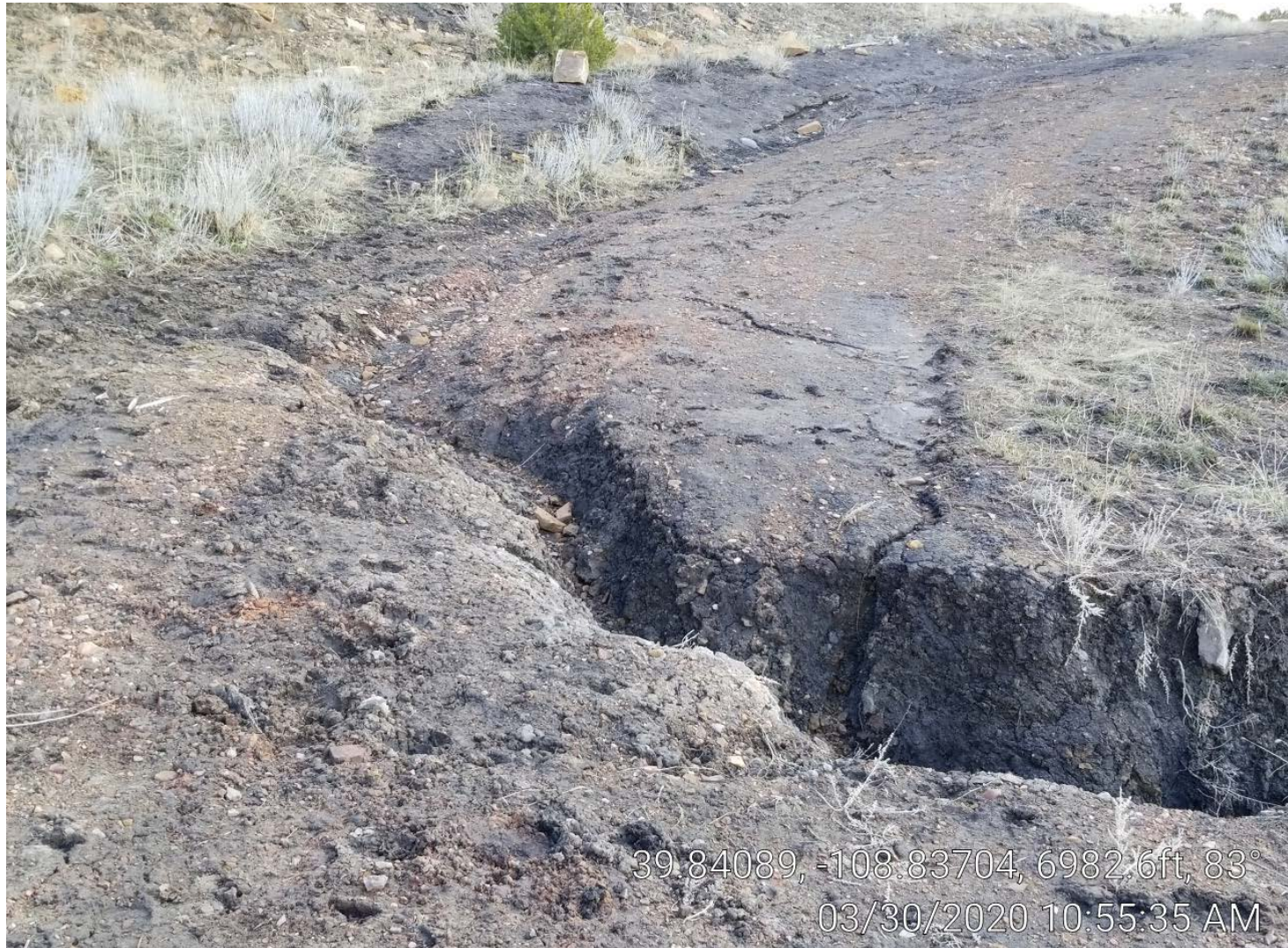
Photo 4. Stormwater channel in lease road.
