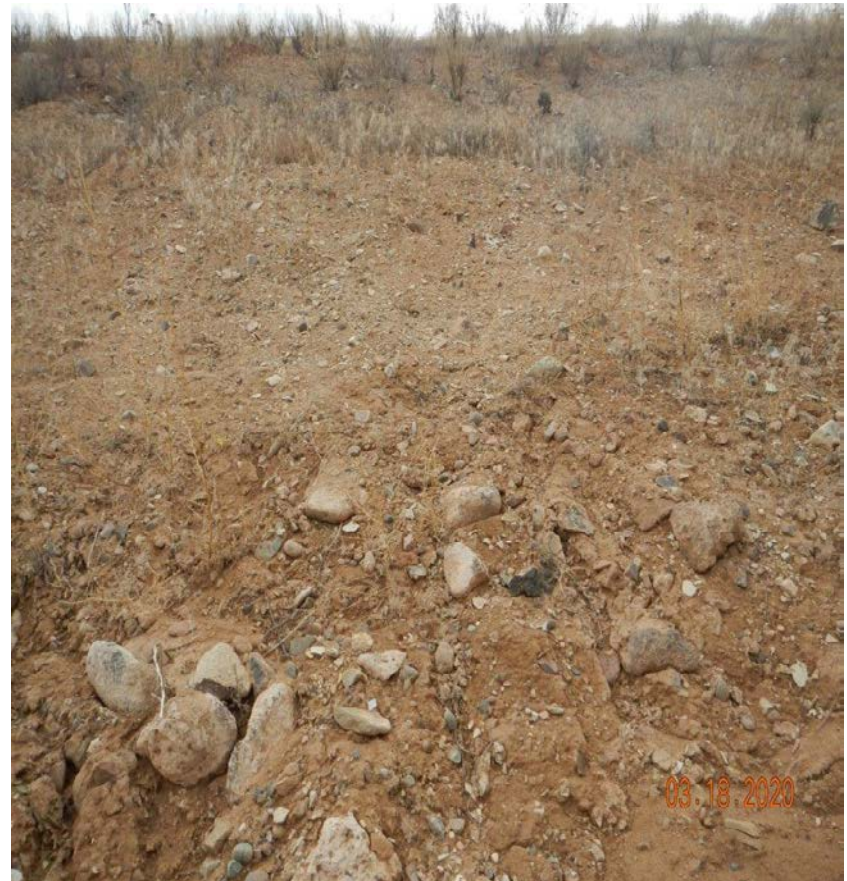
Photo#5: Erosion commencing on Cut Slope.
