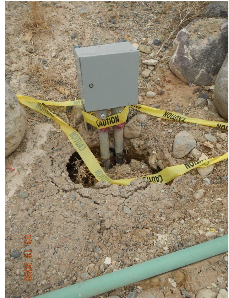
Photo#7: Subsidence at electrical riser..
