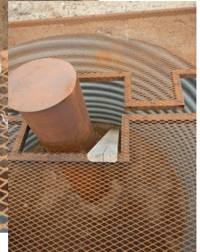
Photo#3: Boards not in position to allow means of Wildlife egress.
