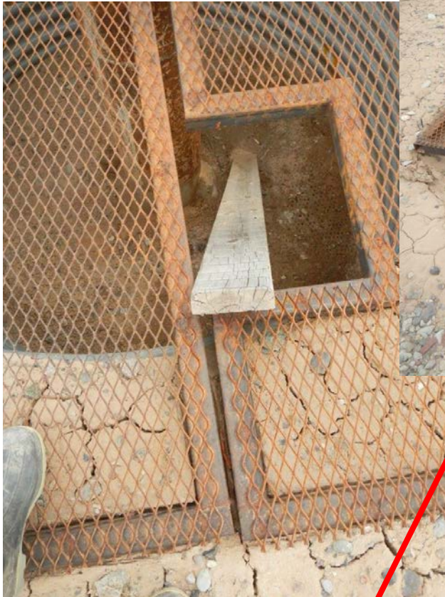
Photo#2: Boards not in position to allow means of Wildlife egress. & Subsidence developing
