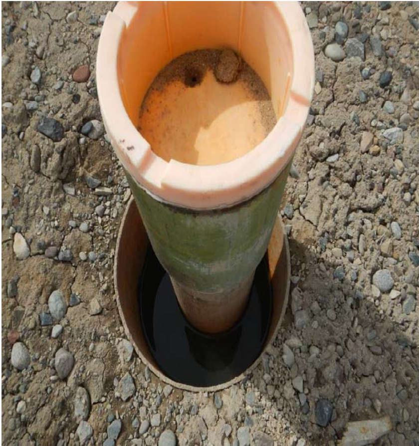
Photo#2: API#045-22340 showing open gap .
