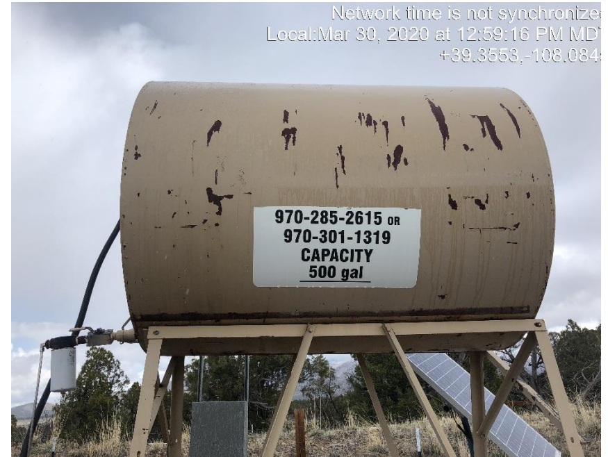
Photo #0872 500 gallon methanol tank missing operator's name.
