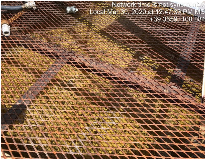
Photo #0871 Oily fluid in Methanol tank containment.
