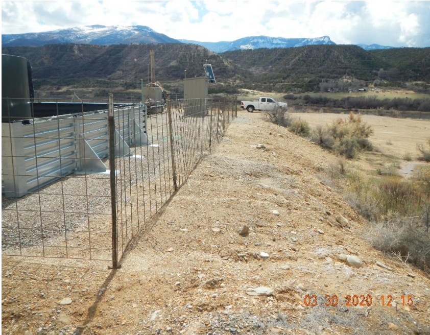
Erosion controls needed behind tank battery.
