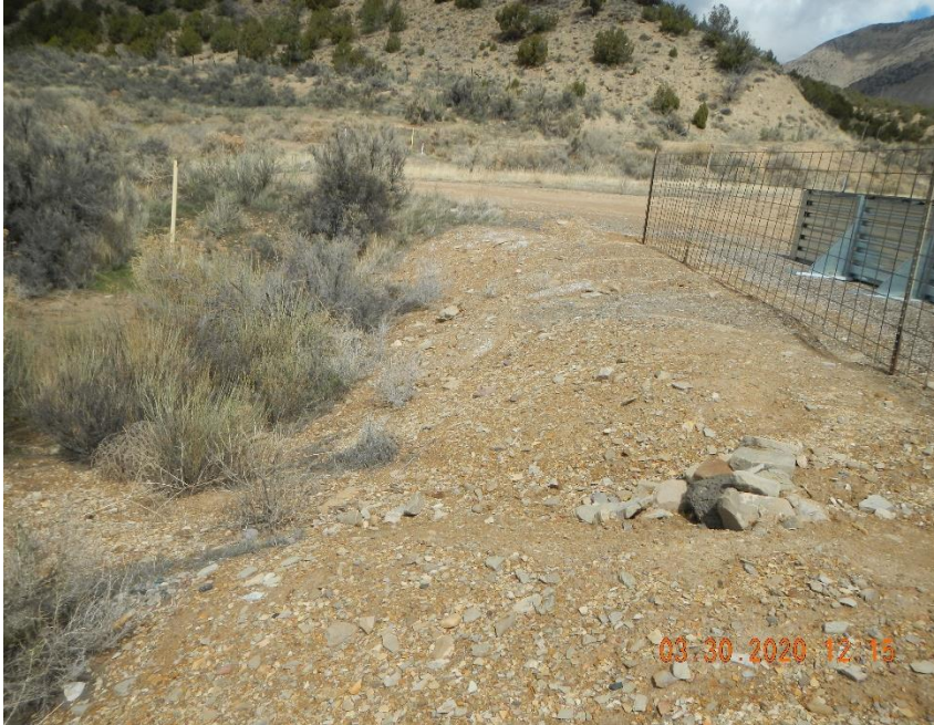
Erosion controls needed behind tank battery.
