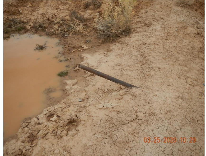
Steel pipe protruding from secondary containment berm.
