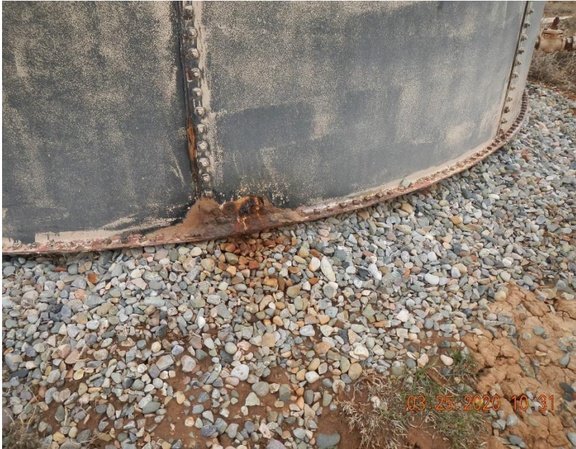
Stained area beneath compromised seam along bottom of AST.
