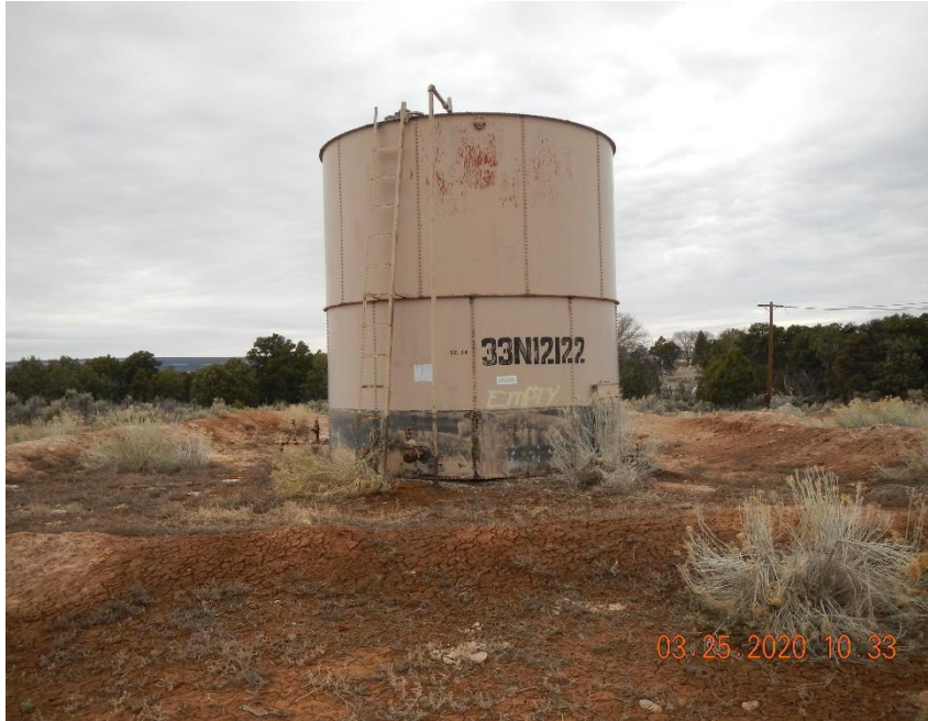
Crude oil AST, marked empty by COGCC field inspector.
