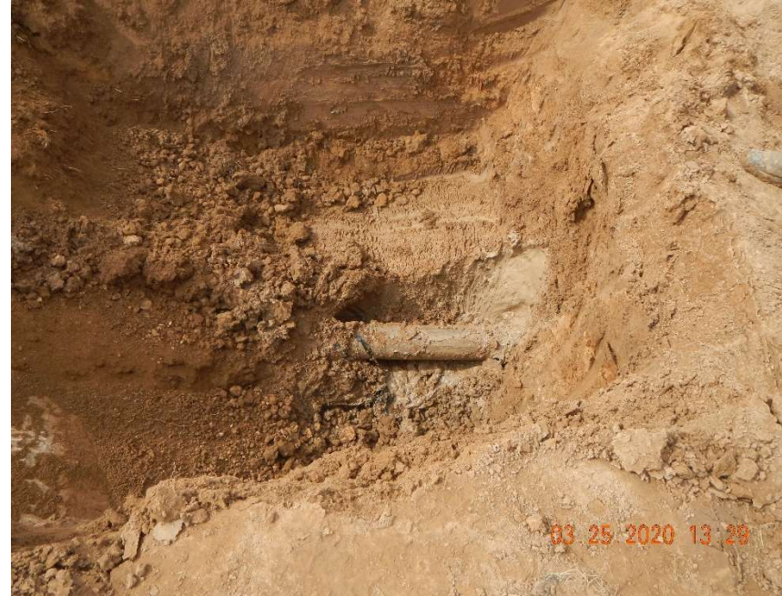
6-inch pipeline excavation, the fluids around the pipeline are from hydrovacing.
