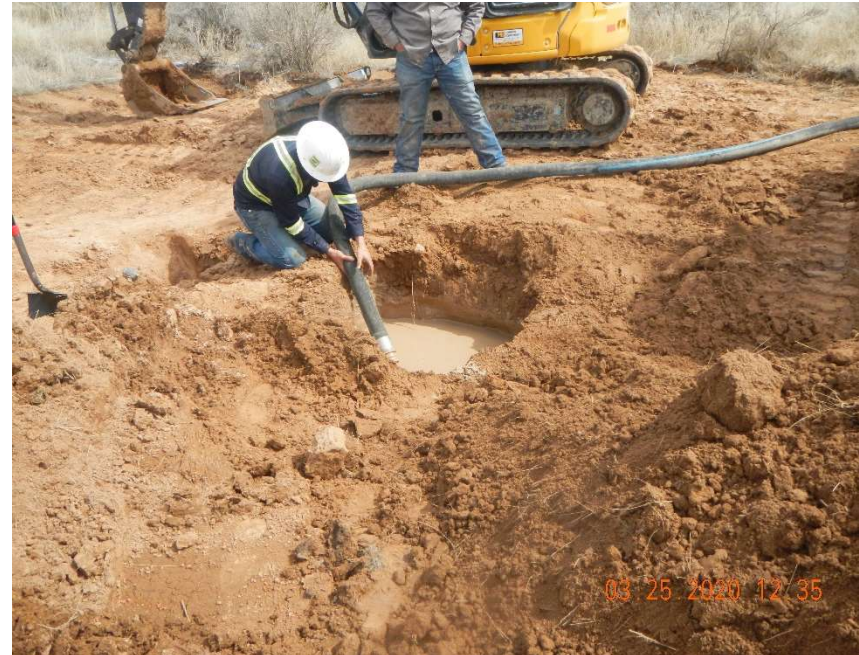
Hydrovacing to located the 6-inch pipeline and the scraped soils around the excavation.
