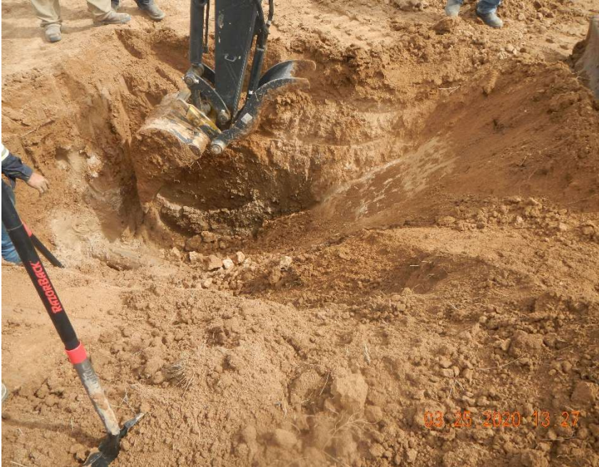
Excavation of the 6-inch pipeline.
