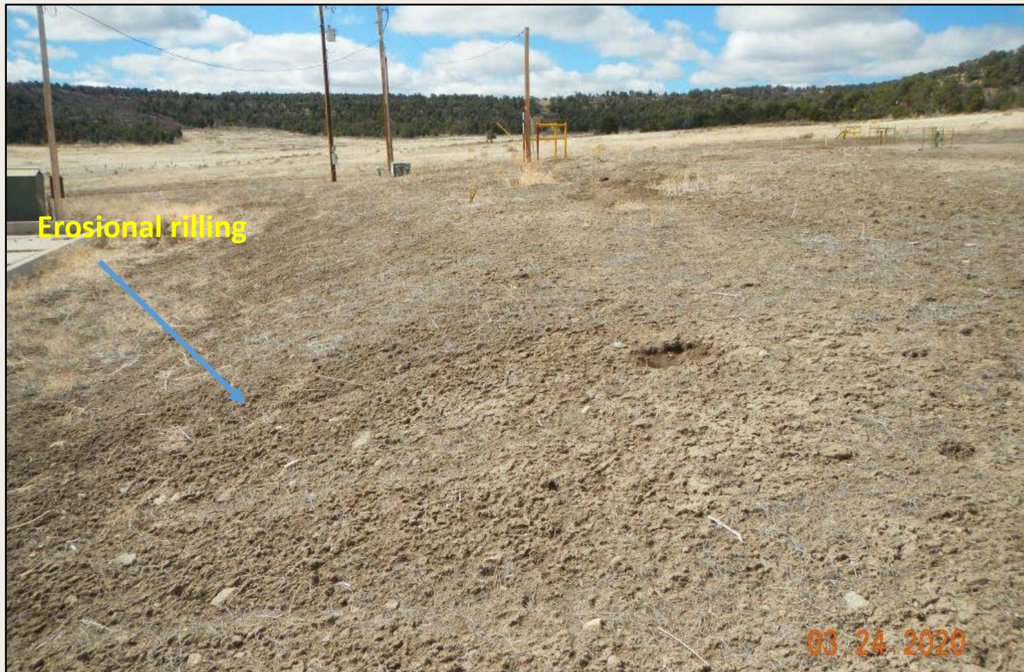
Photo 2. View of the eastern fill slope from the northeastern edge facing southward. Slope is largely comprised of bare soils. Erosional rilling observed along slope.
