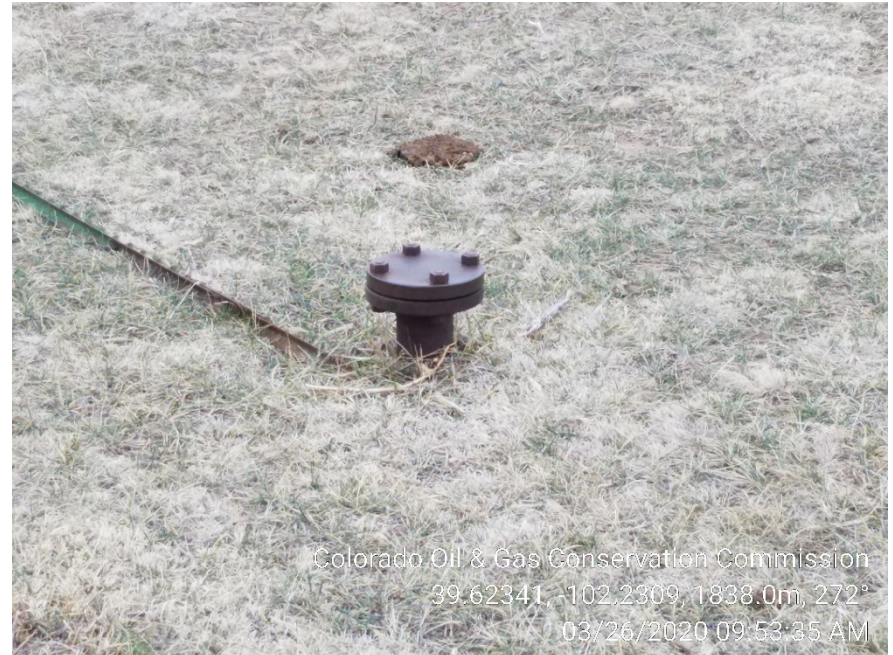
2. Pipeline riser for old meter run.
