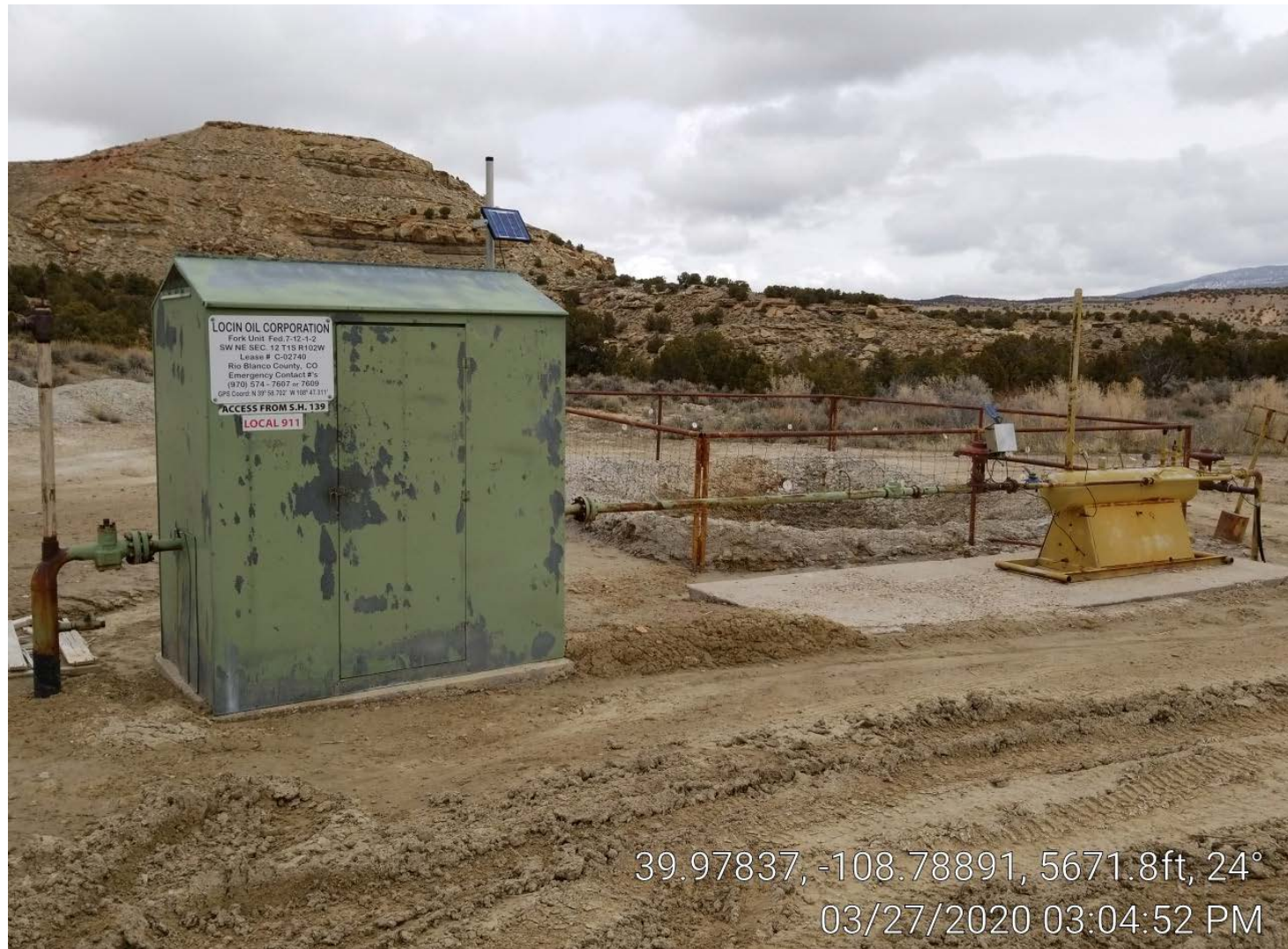
Photo 3. Meter building, separator, and pit.
