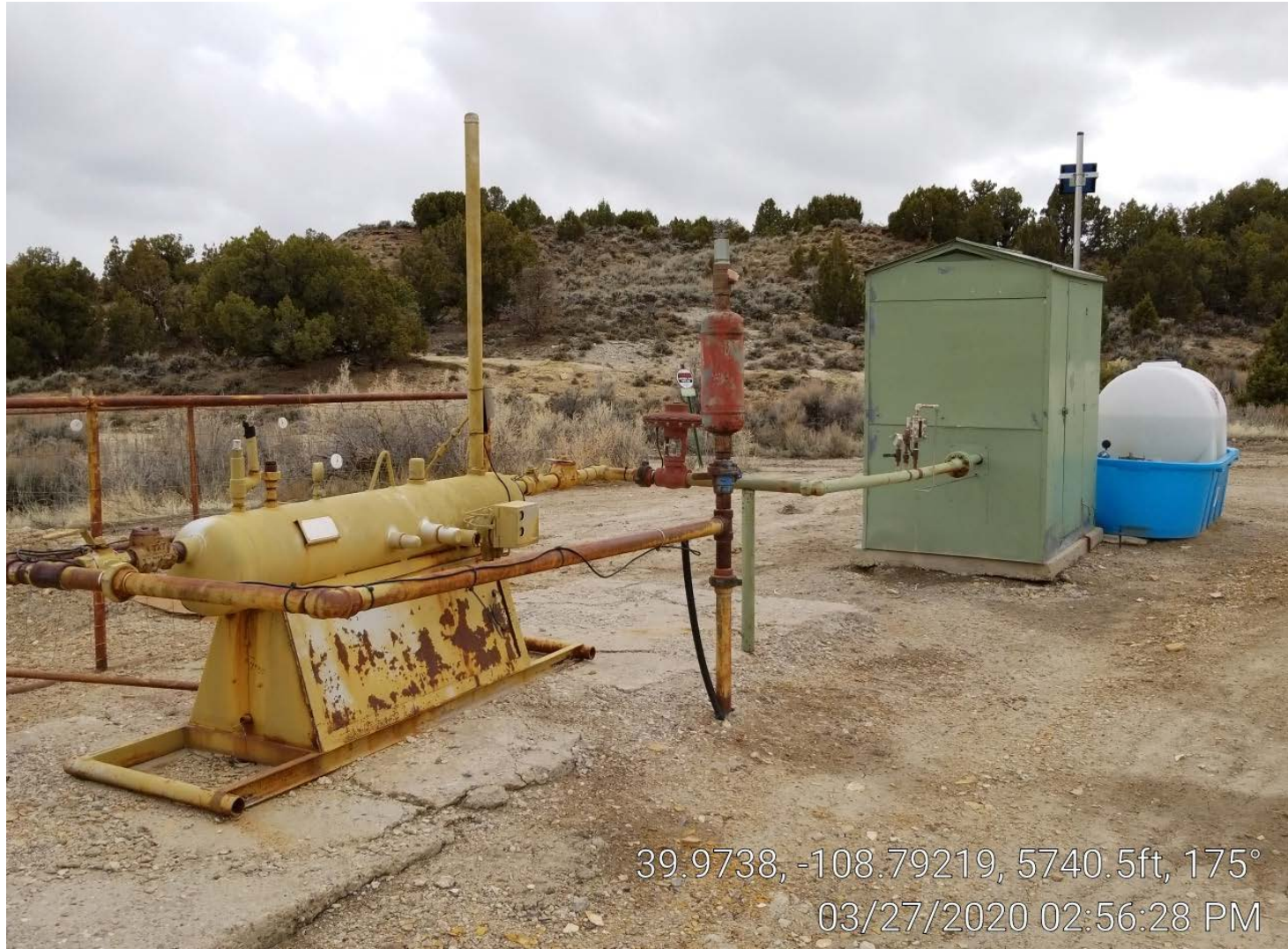
Photo 2. Separator & meter building.
