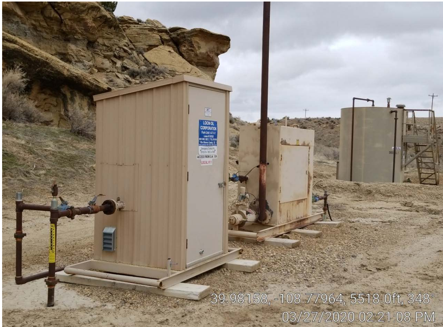
Photo 3. Meter building, separator, and tank.
