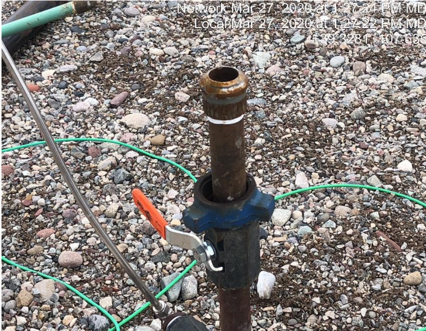
Photo #0863 Flow line risers not LO/TO.
